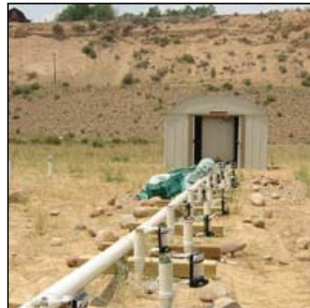
Wells at old Rifle mine inject acetate (vinegar) into the ground to stimulate the growth of microbes already in the soil.
